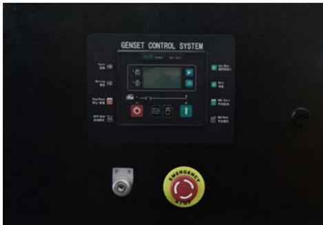
**Baifa Standard Control Panel** uses micro processing technique integrating digital, intelligent and network techniques which can carry out functions including auto start/stop, data measure, alarming. The controller uses LCD display, optional Chinese and English display interface with operation easy and reliable. It can be widely used in all types of generator automatic control system for compact structure, advanced circuits, simple connections and high reliability
